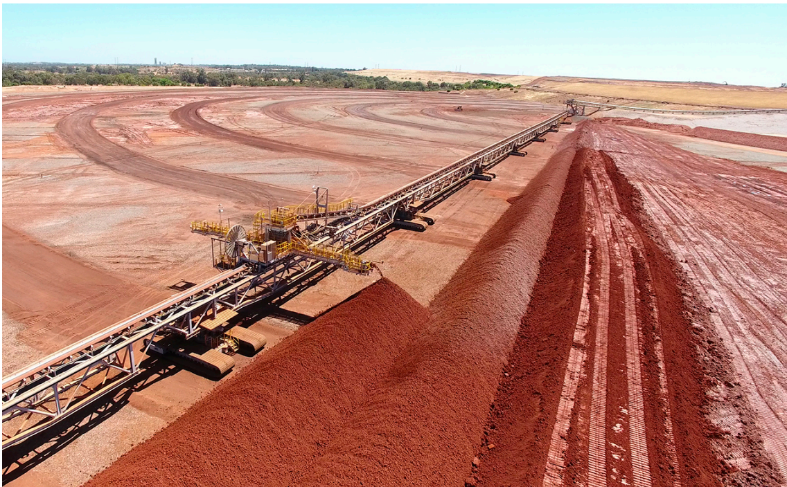
Figure 7. Red mud dry-stacking.
